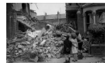
Below: Remains of a house after a bombing raid during the Blitz
